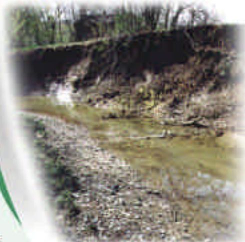
Kinnickinnic River eroding stream bank.
