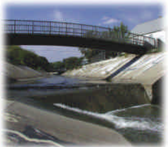
Kinnickinnic River concrete-lined channel, 9th Street.
