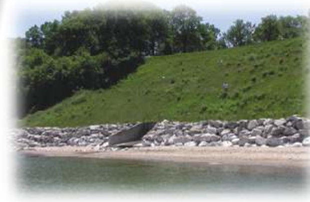
Storm sewer outfall to beach area.
