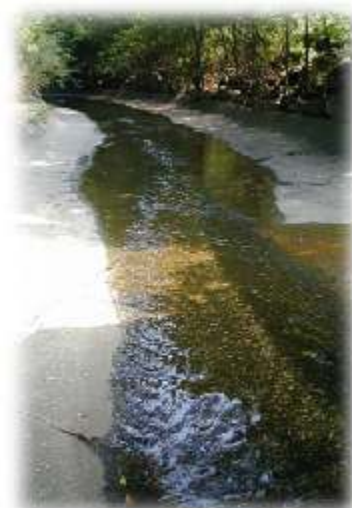
Concrete lined channels
