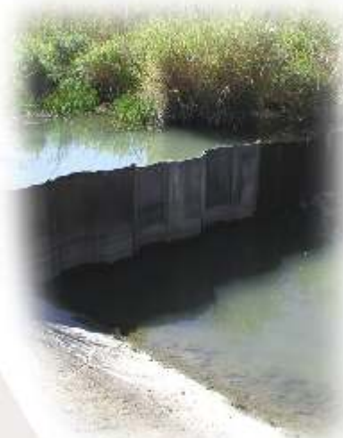
Mainstem of Oak Creek with steel sheet pile weir.
