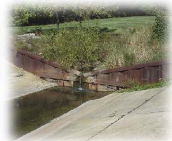
Steel weir on North Branch Oak Creek and concrete channel.
