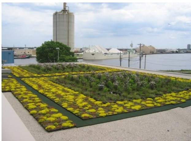
Figure ES-5. Green roof at the GLWI; a demonstration project to highlight strategies for mitigating stormwater runoff.
