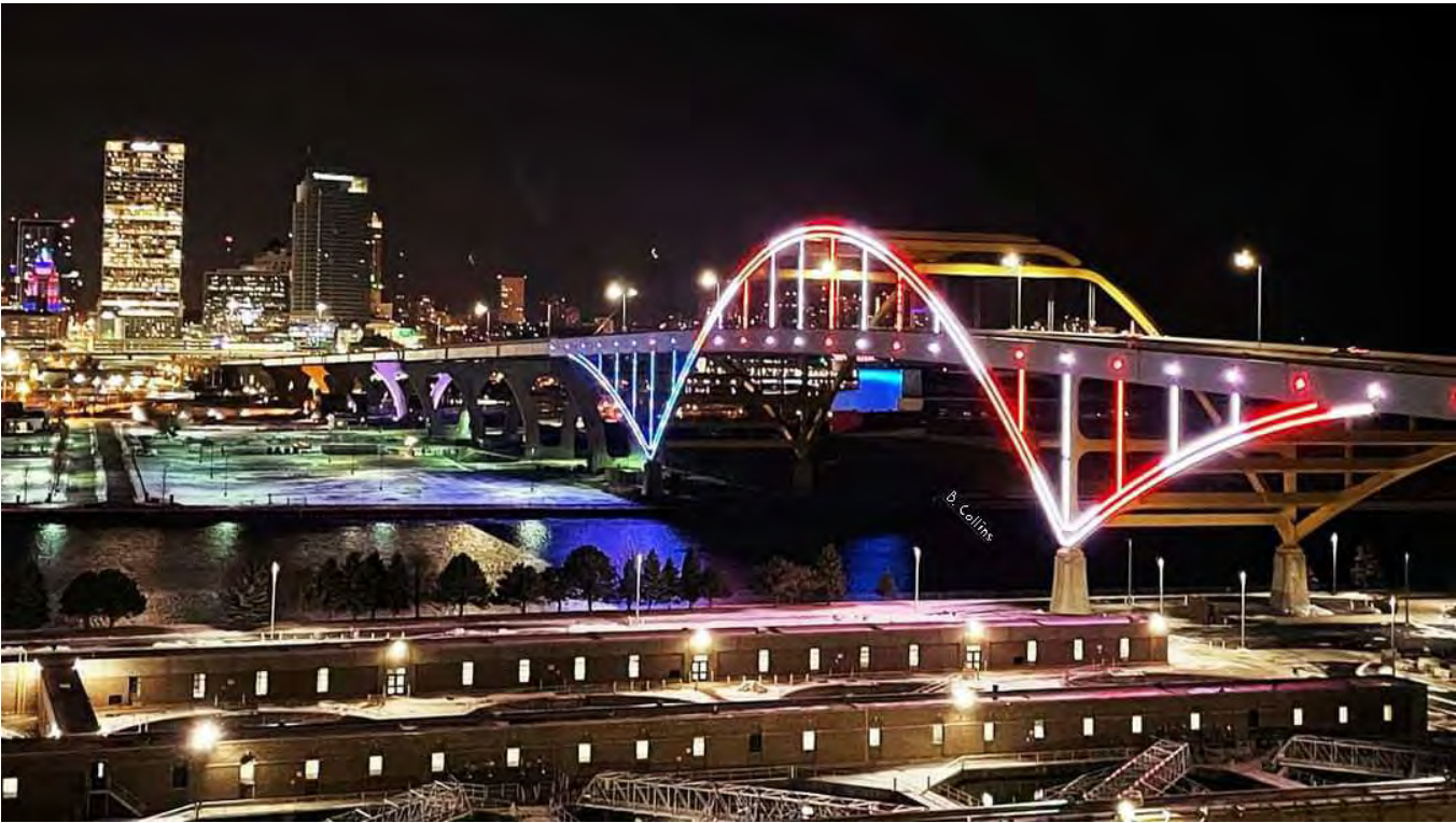
Downtown Milwaukee and the Hoan Bridge as seen from Jones Island.
