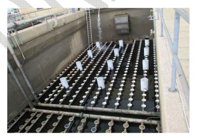
Figure 4: Standard Layout for Large Bubble Low Pressure Air Mixing System in Aeration Basin
