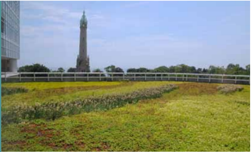
Columbia St. Marys Green Roof
