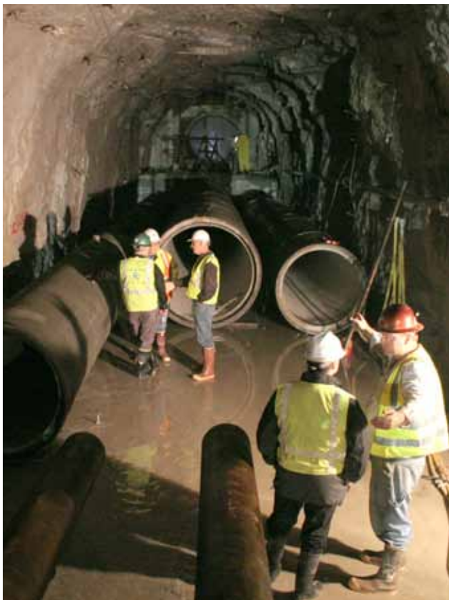
Construction of the Harbor Siphon Tunnel
