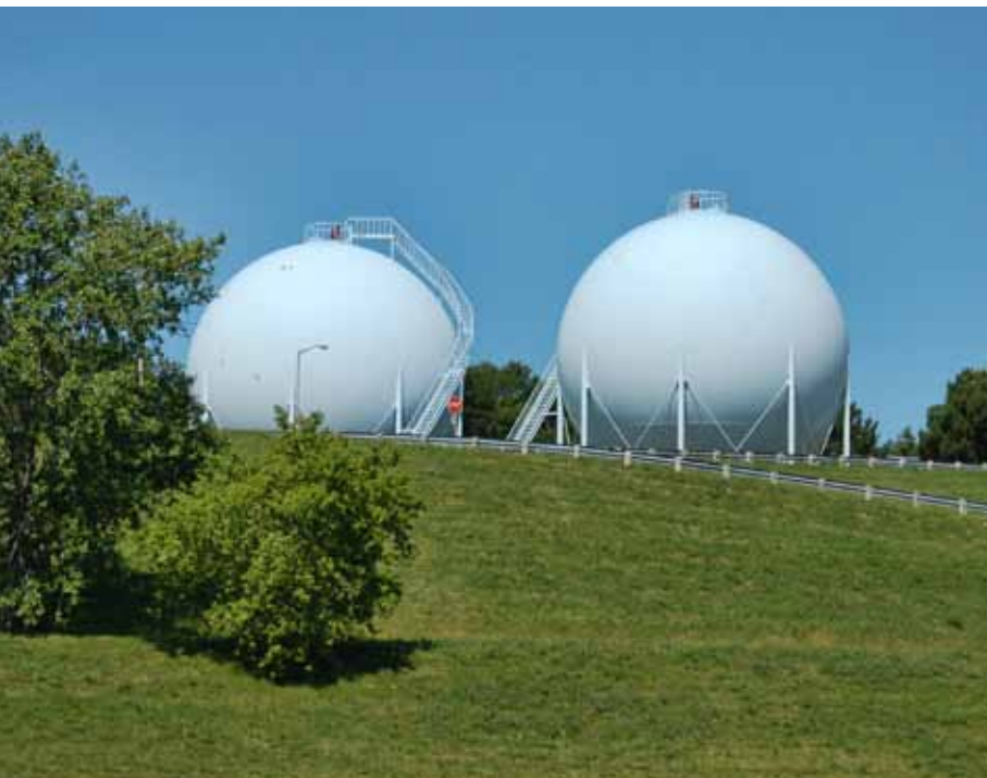
South Shore Water Reclamation Facility Digester Gas Storage Spheres
