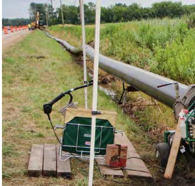
MMSD's Landfill Gas Pipeline Project
