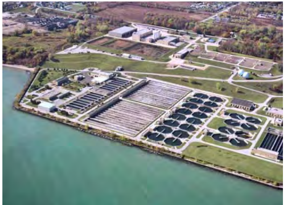
South Shore Water Reclamation Facility
