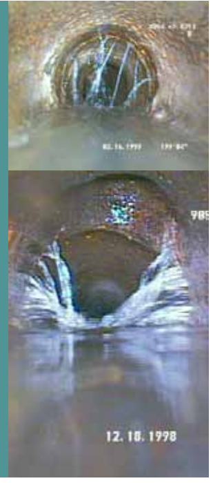
Actual Recorded Inspections
