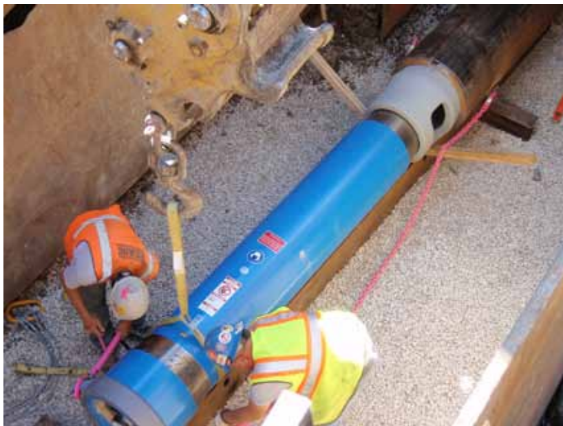
Landfill Gas Pipeline
