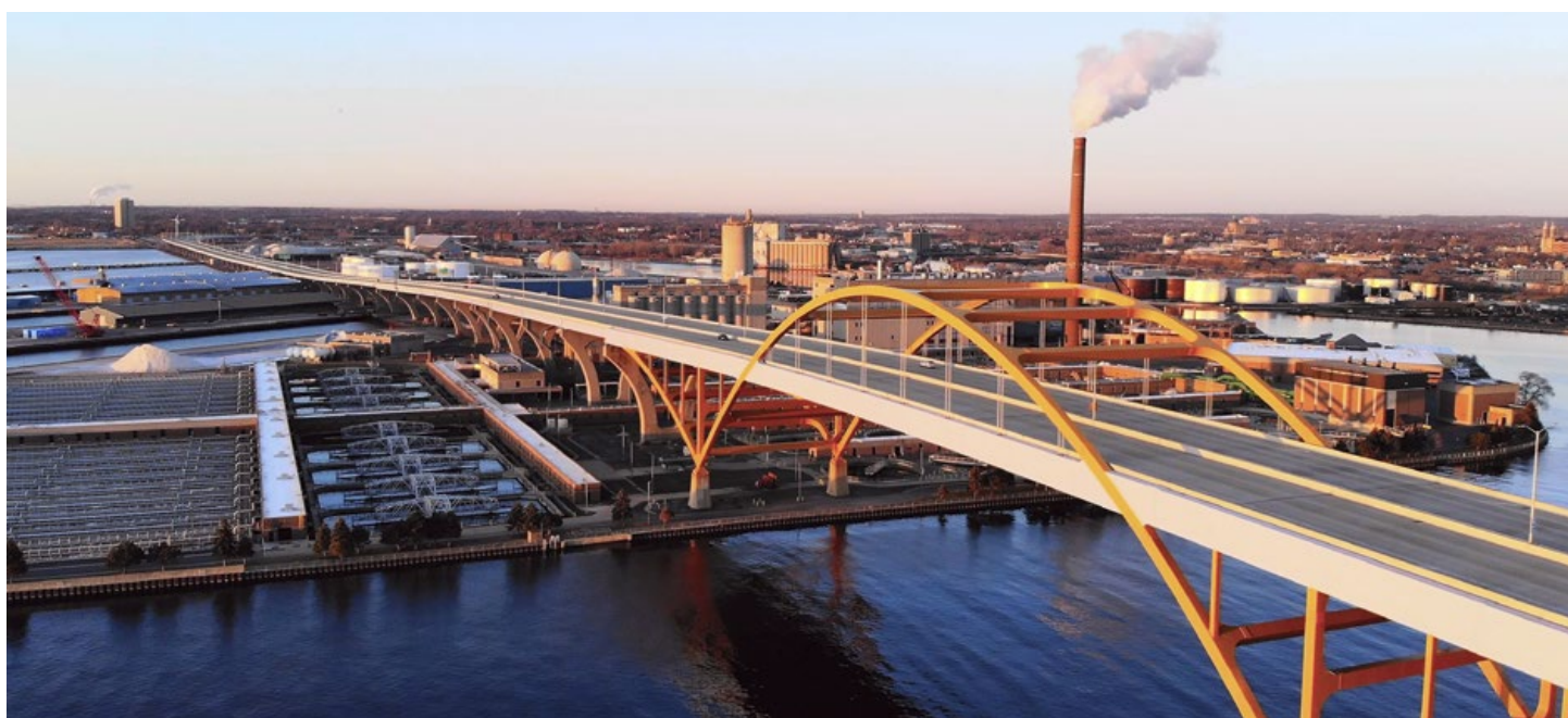
Jones Island Water Reclamation Facility
