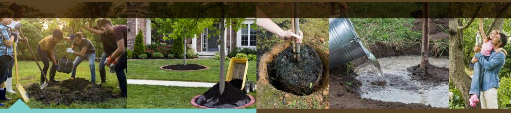
Stormwater trees can hold rainwater on their leaves and branches, infiltrate it into the ground, absorb it through root systems, and evapotranspire it to the atmosphere. They can be planted in engineered soils and used with other types of green infrastructure.
