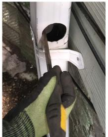
8. Drill hole in downspout using the large hole saw (2-1/8"). File down the sharp edges.
