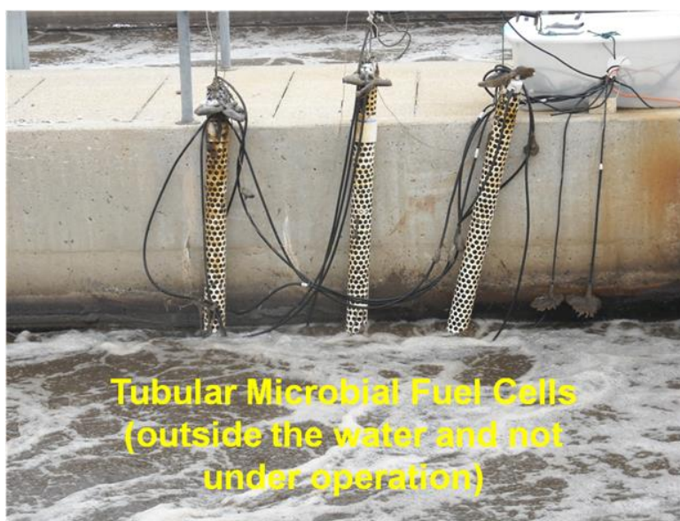
Figure 3.1 MFCs installation in the aeration tank.
