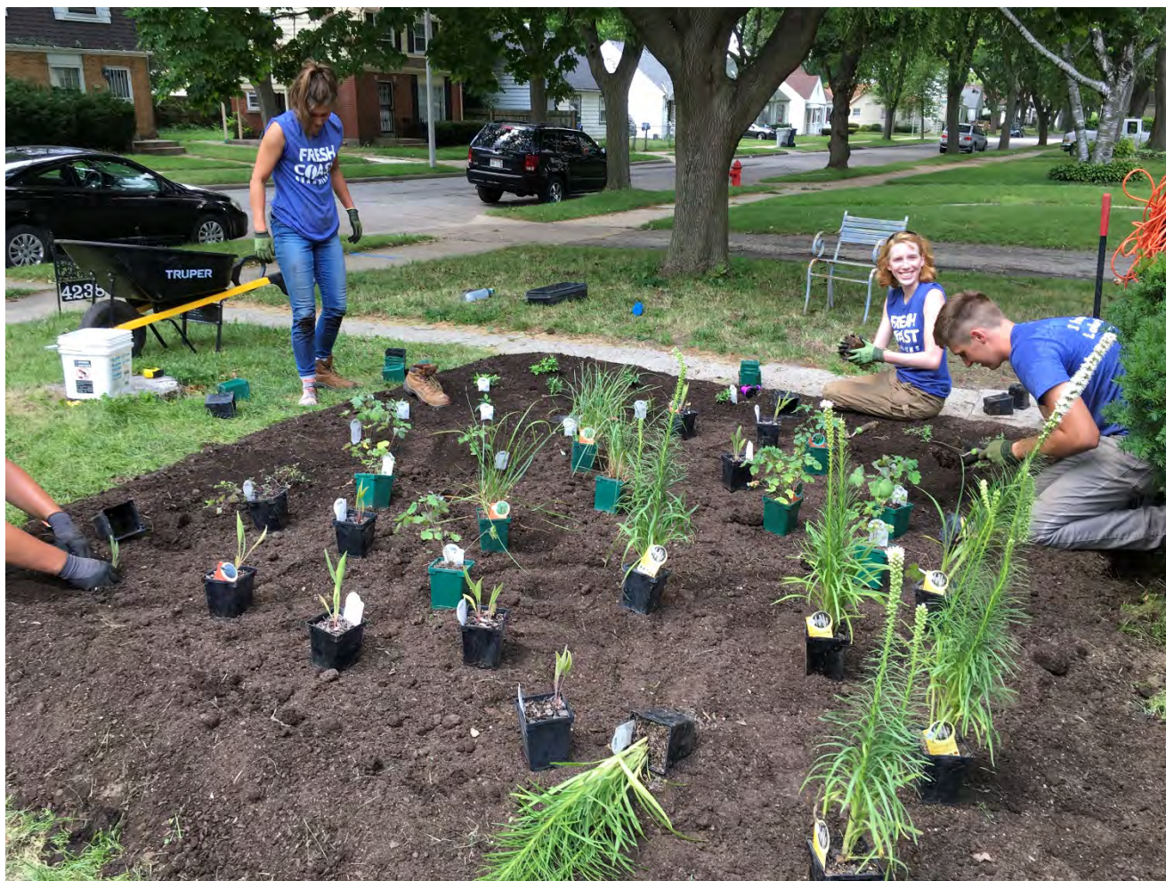
Summer intern students install a rain garden to manage water where it falls.
