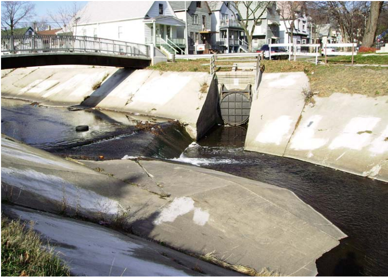
KK River at pedestrian bridge, drop structure, and combined sewer outfall near 8th Street
