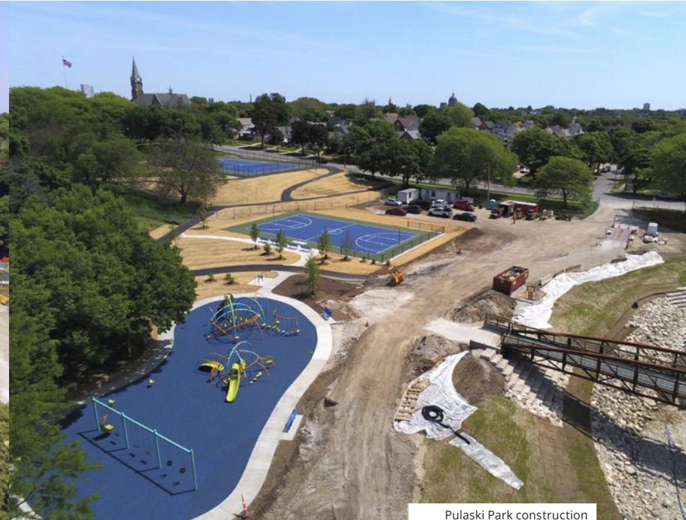
Pulaski Park construction
