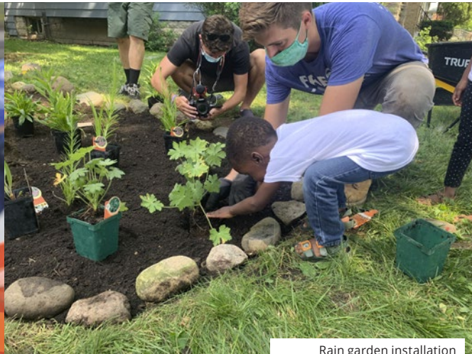
Rain garden installation
