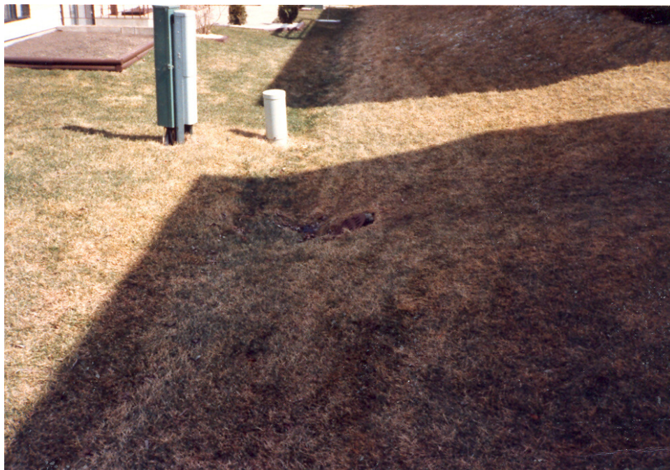
OUTLET PIPE FOR DOWNSPOUT AND CLEAR WATER SUMP SURFACES IN BACKYARD
