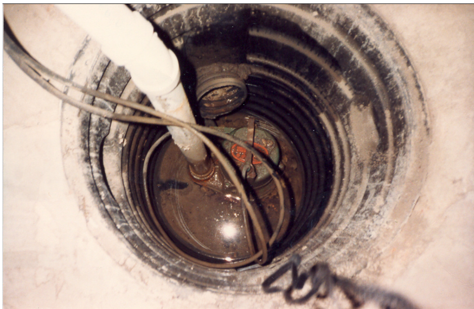
CLEAR WATER CROCK WITH TILE INLET
