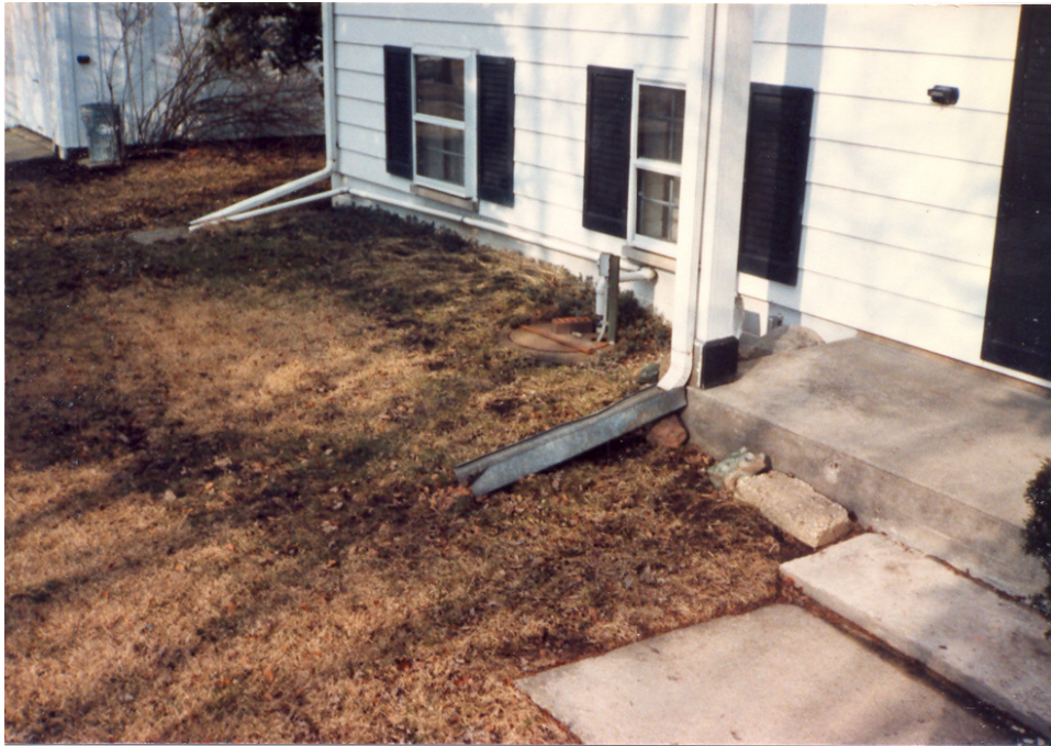
CLEAR WATER SUMP PUMP LOCATED OUTSIDE OF HOME. DISCHARGES MORE THAN 3' FROM WALL
