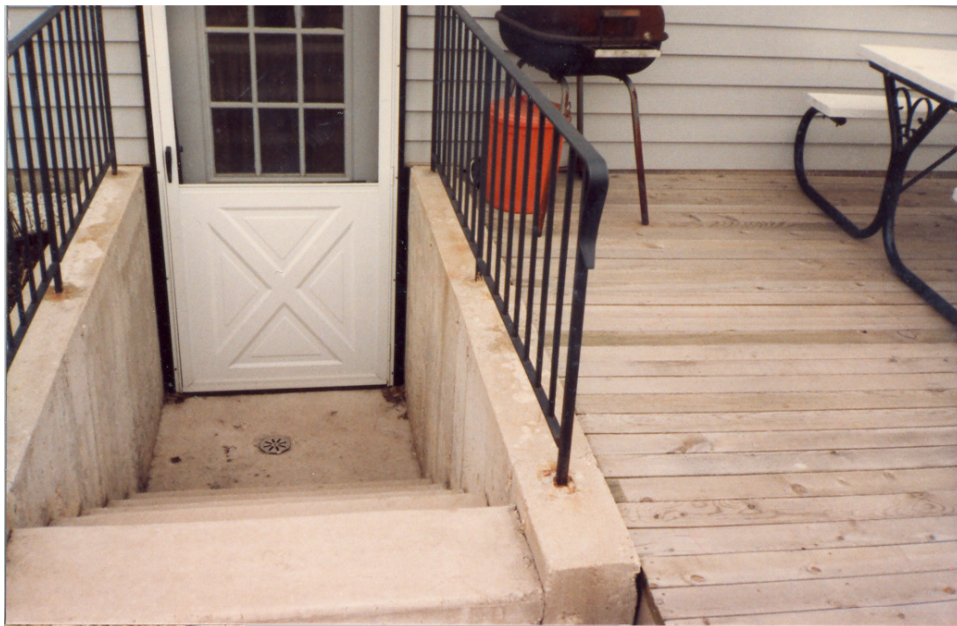
STAIRWELL WITH DRAIN
