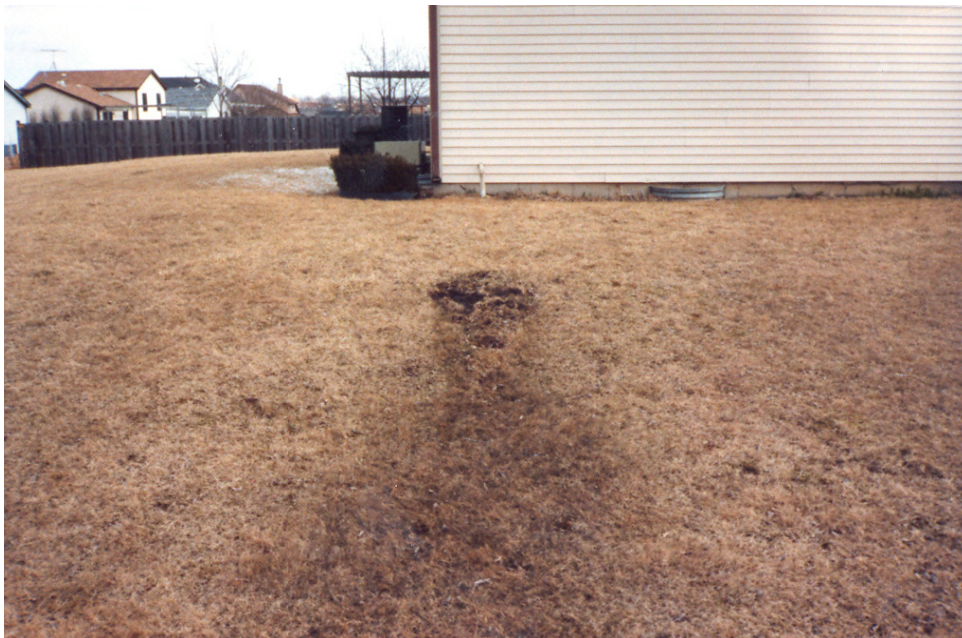
FURTHER INVESTIGATION SHOWS THAT THE OUTLET PIPE DISCHARGES MID-YARD
