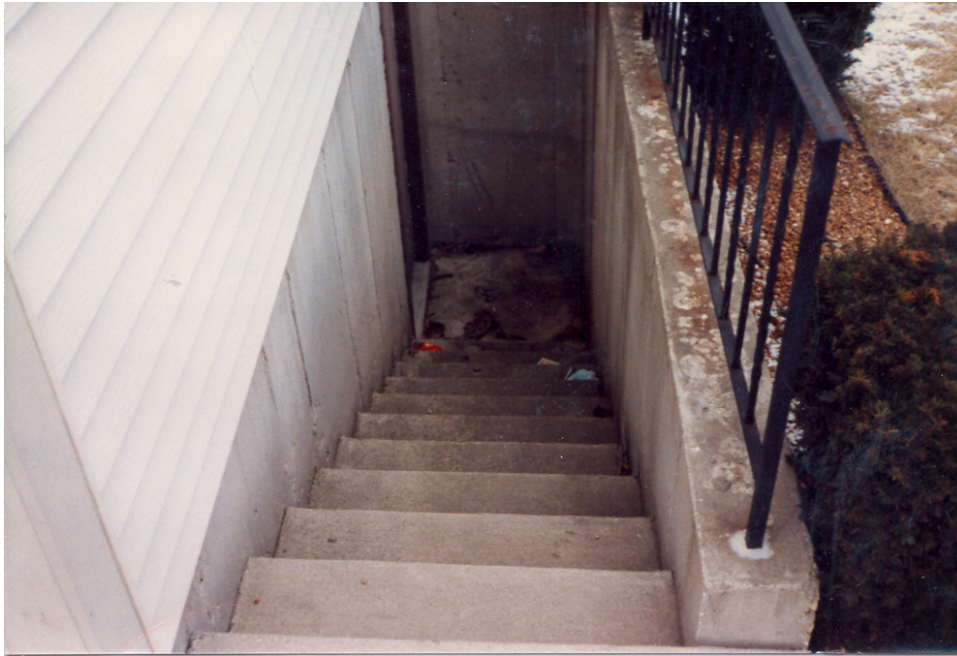
STAIRWELL WITH DRAIN
