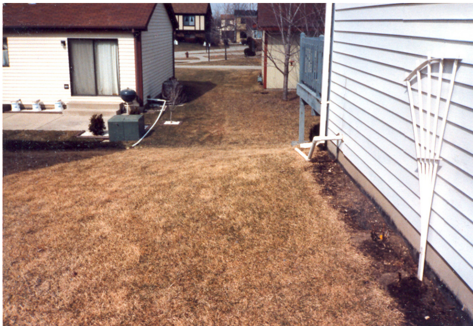
CLEAR WATER SUMP DISCHARGE OUTSIDE – MORE THAN 3' FROM WALL
