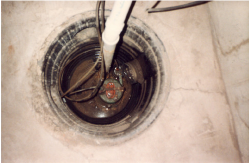
CLEAR WATER CROCK WITH TILE INLET
