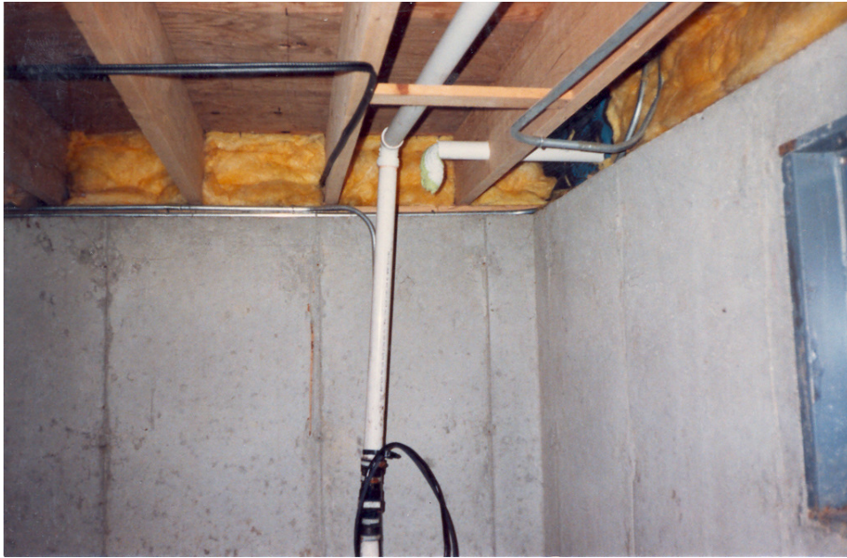
CLEAR WATER SUMP. DISCHARGE TO OUTSIDE DISCONNECTED AND REROUTED.
