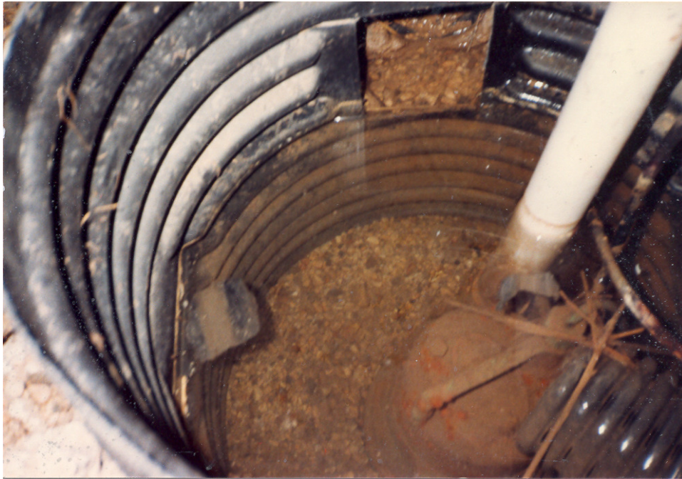
CLEAR WATER CROCK WITH A TILE INLET LOCATED IN CRAWL SPACE
