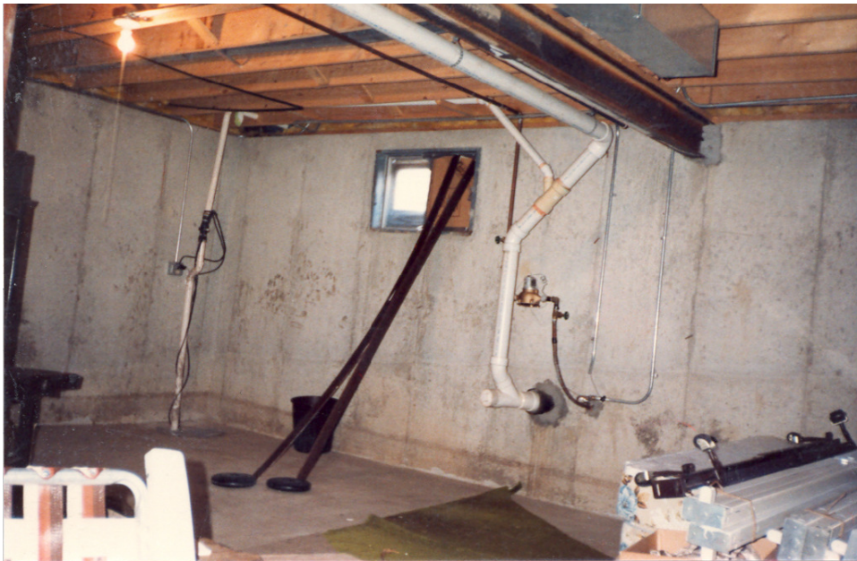
CLEAR WATER SUMP DISCHARGE CONNECTED TO SANITARY SEWER.
