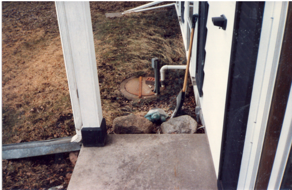
CLEAR WATER SUMP PUMP LOCATED OUTSIDE OF HOME. DISCHARGES MORE THAN 3' FROM WALL
