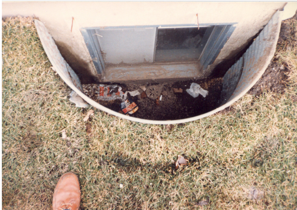
WINDOW WELL WITH DRAIN
