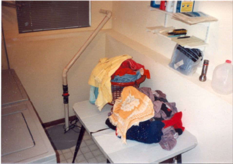
CLEAR WATER CROCK LOCATED IN A UTILITY ROOM OF A BI-LEVEL HOME
