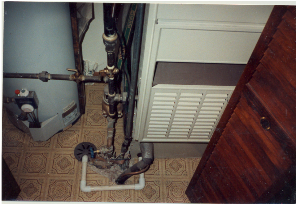
FLOOR DRAINS ARE USUALLY LOCATED NEAR UTILITIES AND/OR LAUNDRY FACILITIES
