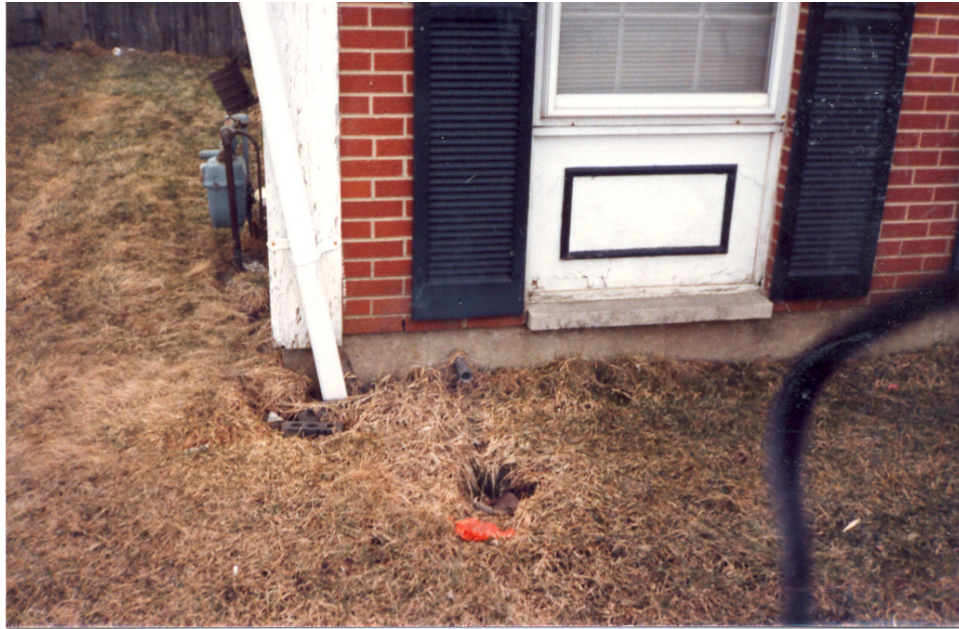
CLEAR WATER SUMP DISCHARGE OUTSIDE – WITHIN 3' OF WALL
