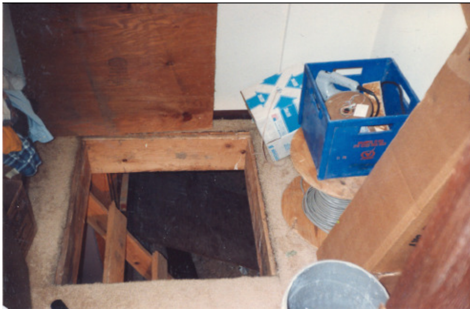
ACCESS INTO A CRAWL SPACE
