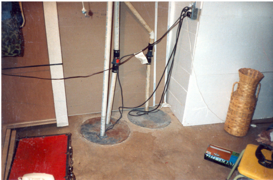
A WASTE CROCK AND A CLEAR WATER CROCK
