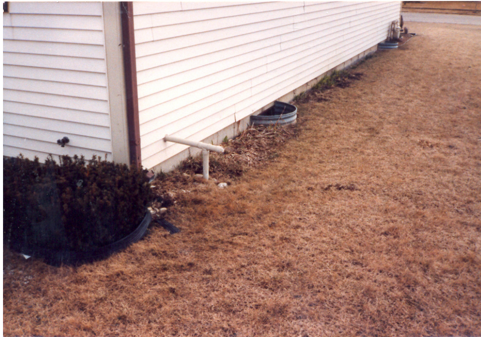
CLEAR WATER SUMP DISCHARGE APPEARS TO GO UNDERGROUND. NOTE 90° BEND IN OUTLET PIPE
