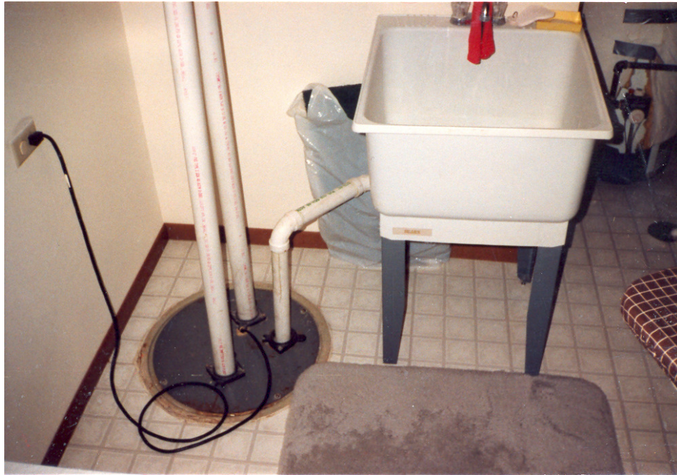
WASTE CROCK THAT TAKES IN STATIONARY TUB AND FLOOR DRAIN
