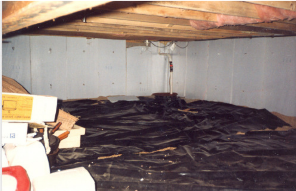
CRAWL SPACE WITH A CLEAR WATER SUMP PUMP
