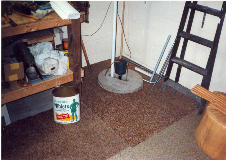
THIS BASEMENT HAS A CLEARWATER SUMP IN ADDITION TO A WASTE CROCK
