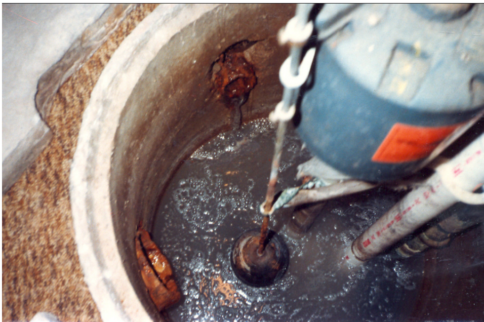
CLOSEUP OF WASTE CROCK SHOWS INLET FOR SHOWER AND FLOOR DRAIN
