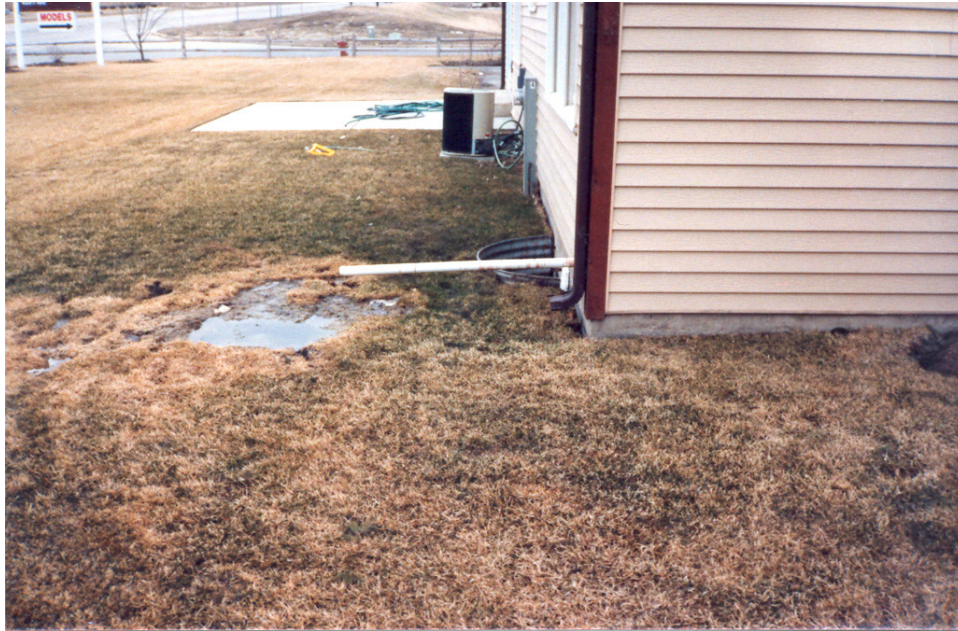
CLEAR WATER SUMP DISCHARGE OUTSIDE – MORE THAN 3' FROM WALL
