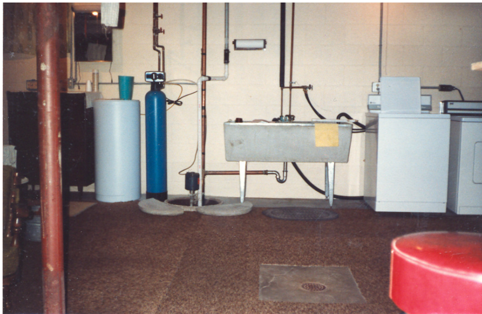
WASTE CROCK TAKES IN LAUNDRY, FLOOR DRAIN, AND SHOWER
