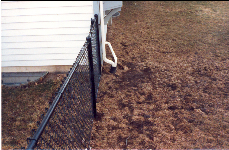
DOWNSPOUT AND SUMP PUMP OUTLET TIED TOGETHER
