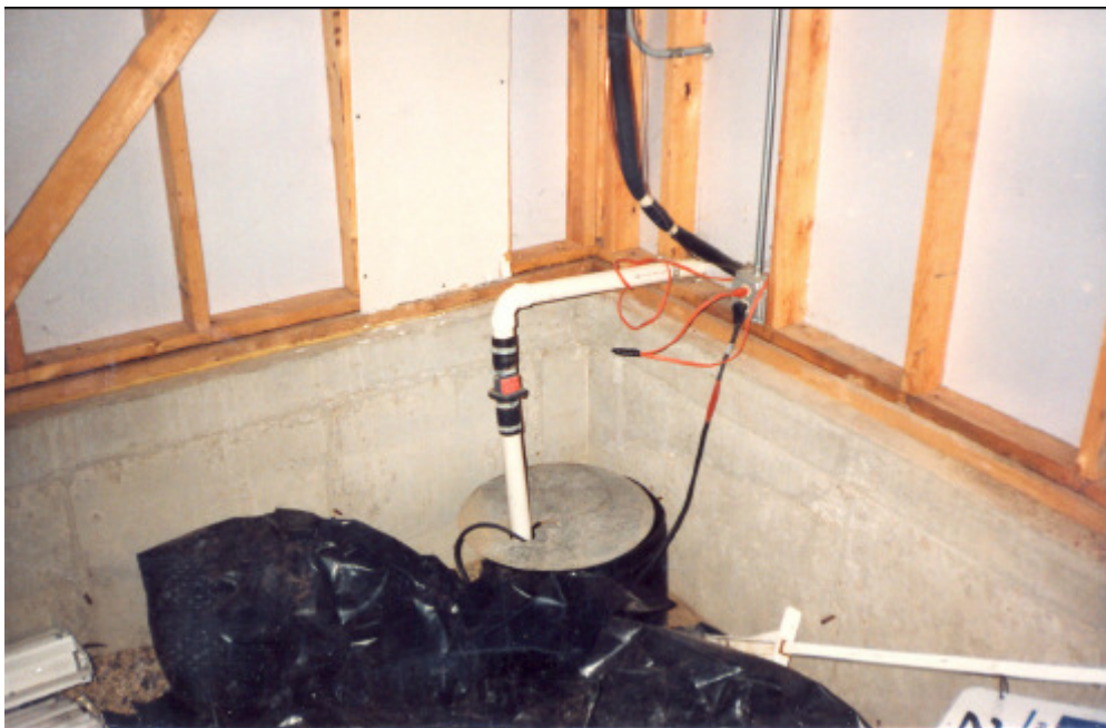
CLEAR WATER CROCK COLLECTS GROUNDWATER SEEPAGE
