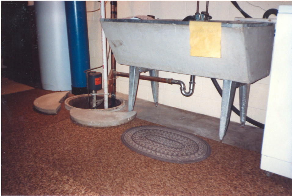
CLOSEUP OF WASTE CROCK SHOWS PLUMBING FOR LAUNDRY DRAINING INTO IT
