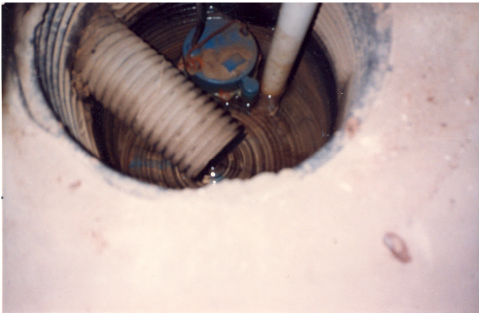
CLEAR WATER CROCK WITH TILE INLET
