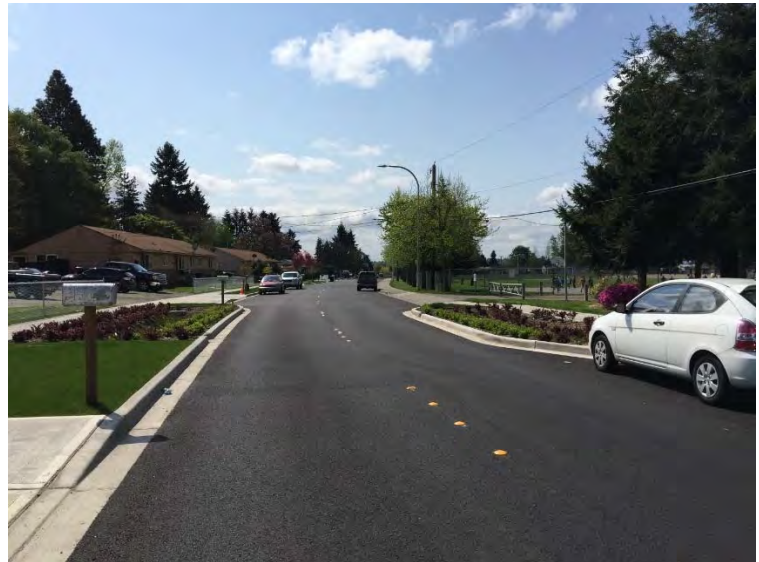
Residential setting bioretention with curb bump outs.
