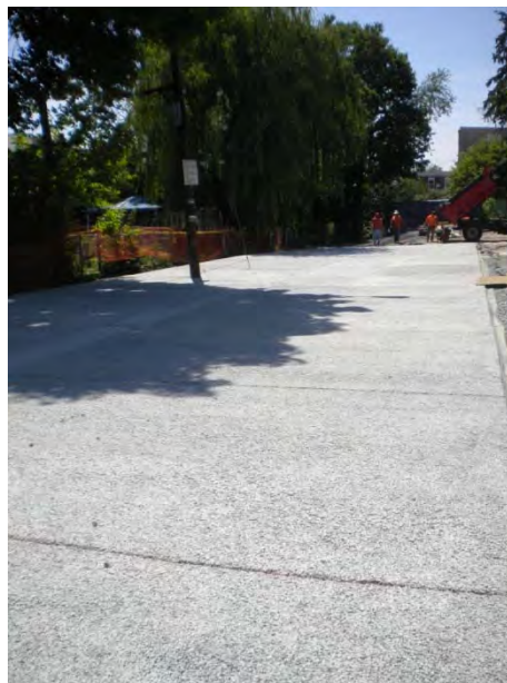
Parking lot with porous pavement and bioretention.
