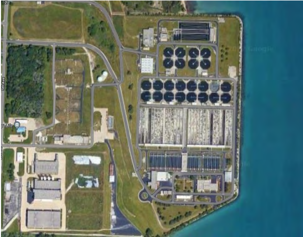
Figure 1-1: SSWRF Aerial Photo
