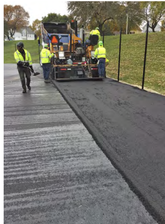
Pervious pavement Installation
