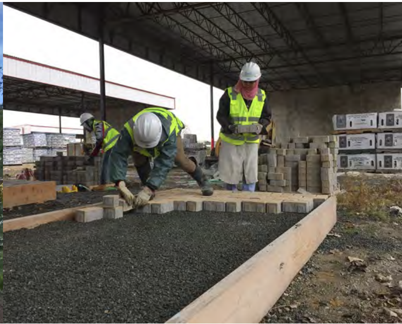
Pervious paver install
