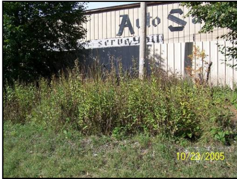
Figure 3. Roof runoff was never diverted to this garden at Seven Stars Auto Salvage in Milwaukee, and the lack of water limited the plant growth.
