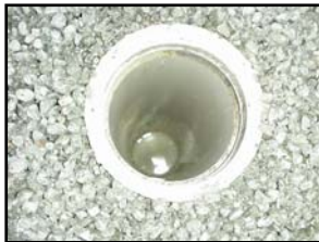
Figure 14. Pervious pavement monitoring port.
