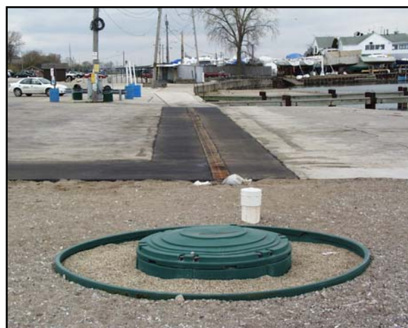
Figure 38. StormTreat device at South Shore Beach.
