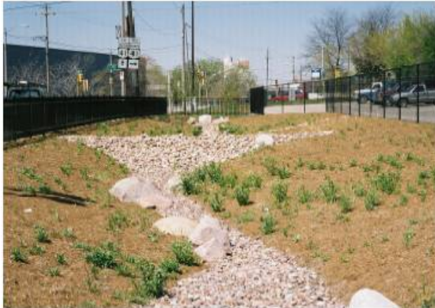
Figure 18. Rain garden and swale following planting.
