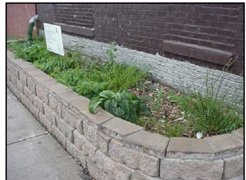
Figure 4. This very small rain garden at Brand Auto has stunted plant growth.
