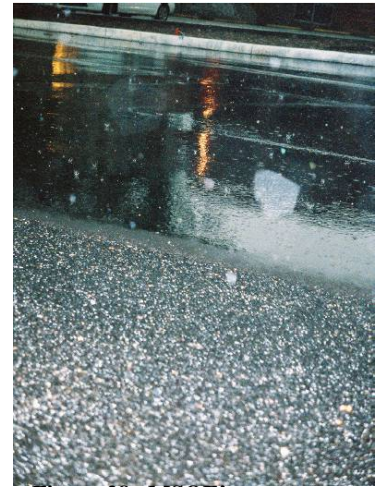
Figure 28. MSOE's porous pavement during a rain event.
