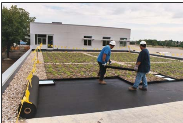
Figure 24. Installation of the zoo's green roof.
