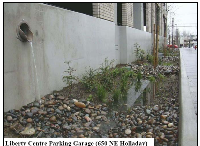
Figure 43. Stormwater Planter (Portland BES).
