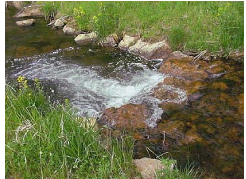
Boulder weir and pool, with narrowed stream to increase velocity over the weir (courtesy of Vernon County Land and Water Conservation Department)
