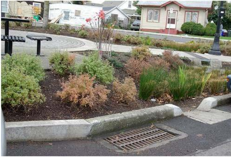
Direct stormwater runoff from streets and parking lots into planting beds designed to filter solids, metals, and other pollutants and infiltrate water to reduce runoff volumes and peak flows
