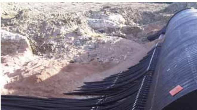
Connecting line at distribution shaft in horizontal design
