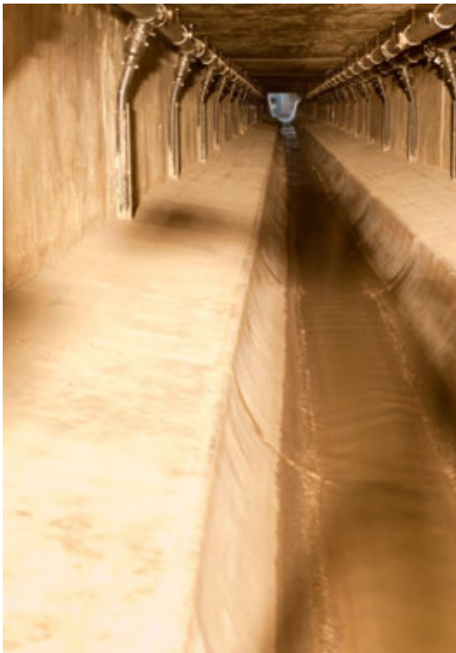
Insertion into existing sewer
