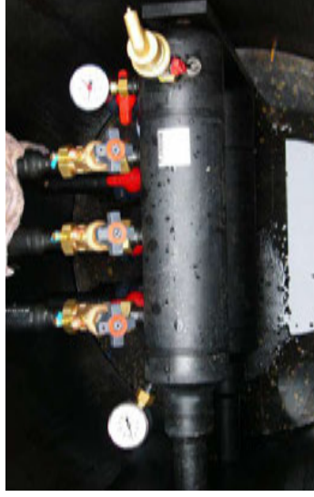
Modular plastic brine manifold inside the manhole
