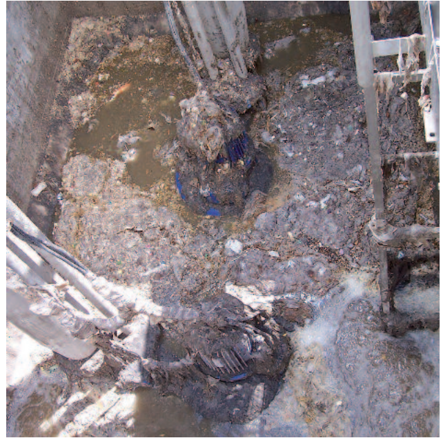
Clogged pumps caused by the solids within the medium to be delivered
