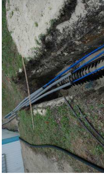
PKS-Thermopipe covered with sand in the trench
